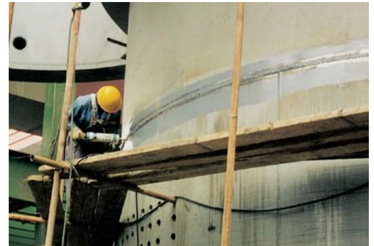
Application of Ultrasonic peening on the vessel
