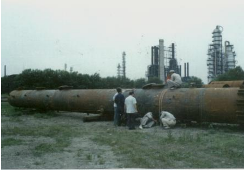
催化裂化装置反应塔爆炸处理 Explosive treatment of reactors for the catalyse-cracking facility
